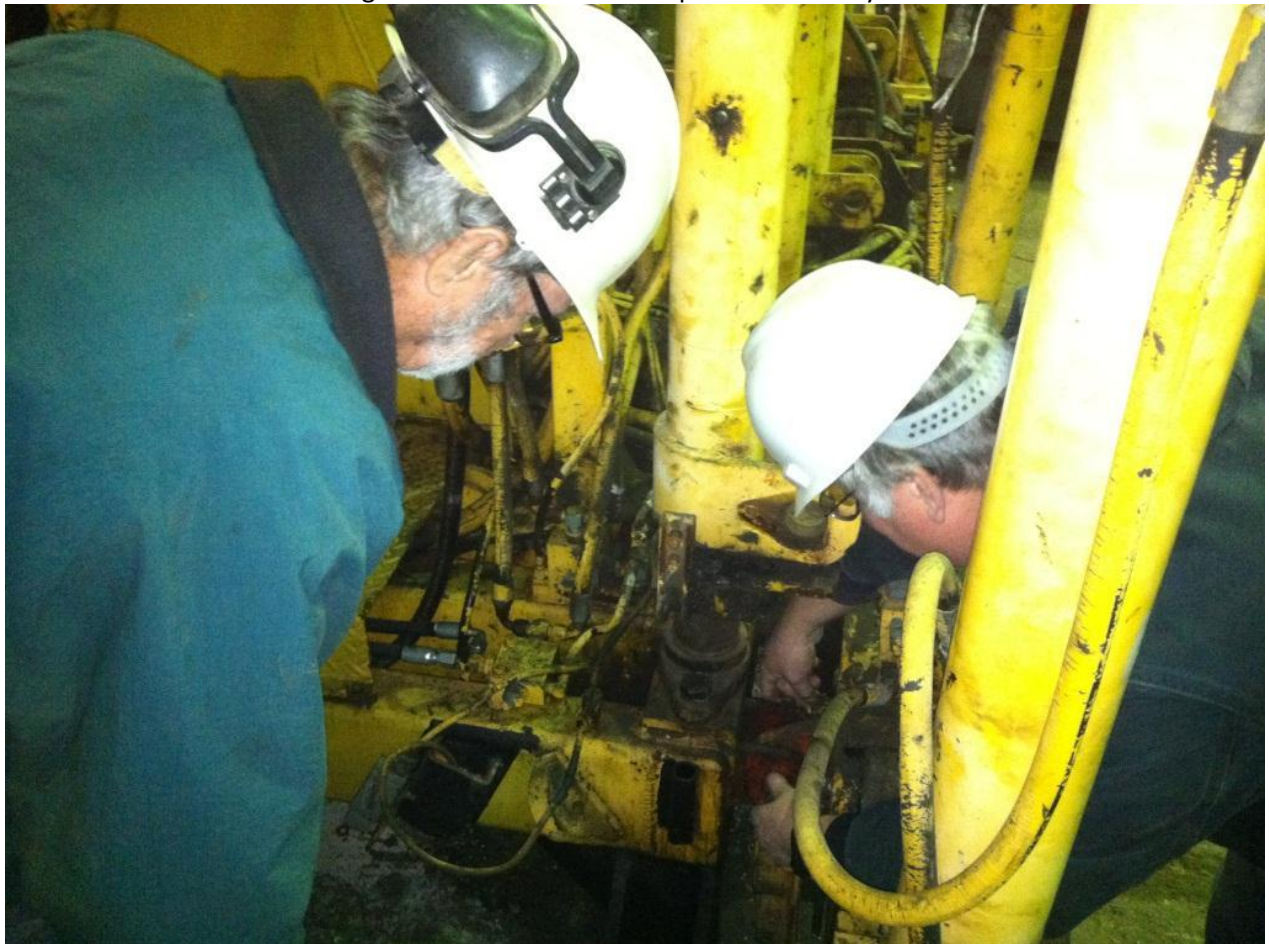
Alan and Chris work on the "new-old" tamper's jacking system
